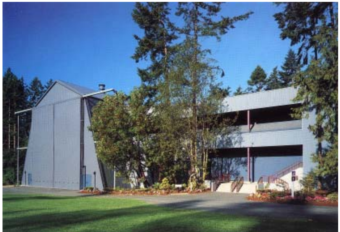
Ft. Worden Balloon Hangar, Port Townsend, Washington, 2001. McCurdy Pavillion/Littlefield Green. (Michael Shopenn)
