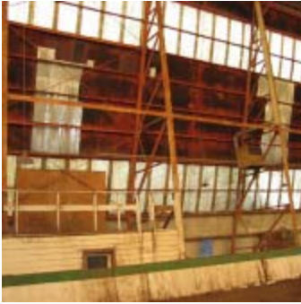
The north elevation of the Balloon Hangar showing the existing 15' x 20' opening and the two tiers of corrugated glass fiber sheets. (Jane Lehman, 2002)
