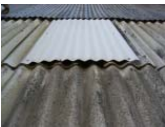
The three ventilators on the roof lean at different angles. (John Martini, 2004)
