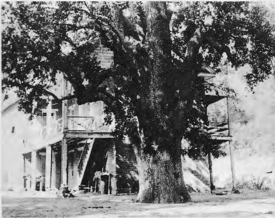
Hospital Building looking west. Circa 1888.
