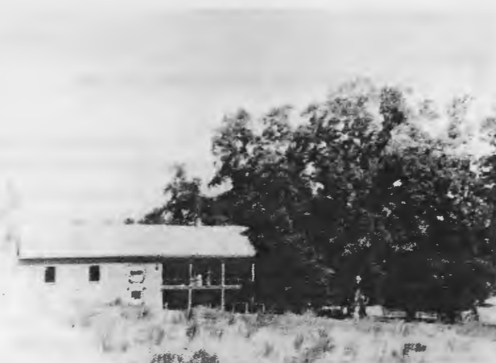
Hospital Building showing missing roof over southwest end of structure. Circa 1888.
