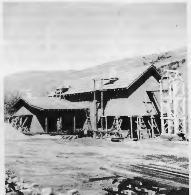
Reconstruction of Officers Quarters almost complete, circa 1957.
