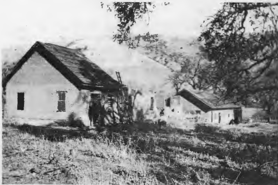
Barracks Building No. 2 showing southwestern end after being converted into a Blacksmith's Shop during ranch period.
