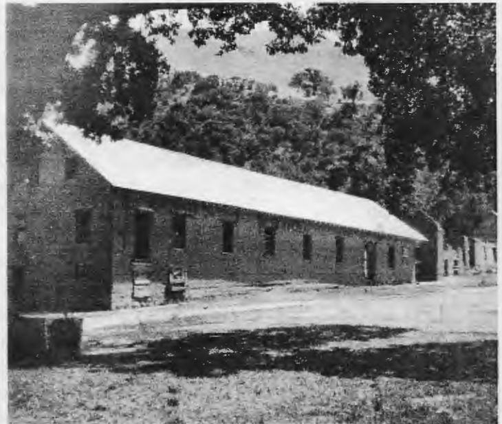
Barracks Building No. 1. Photo circa 1888.
