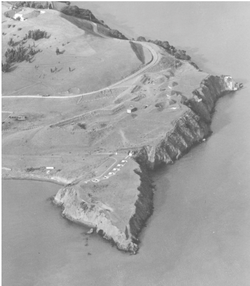
This enlargement of a 1925 aerial photo of Fort Baker clearly shows Point Cavallo, Battery Yates, and the earthworks of Battery Cavallo. Visible within the battery is the flat-roofed powerhouse for Batteries Yates/Duncan and Searchlight #11. On the hill to the left is Battery Duncan.(Courtesy Golden Gate National Recreation Area, Park Archives, GOGA-1766, Lloyd 30th Infantry Album.)
