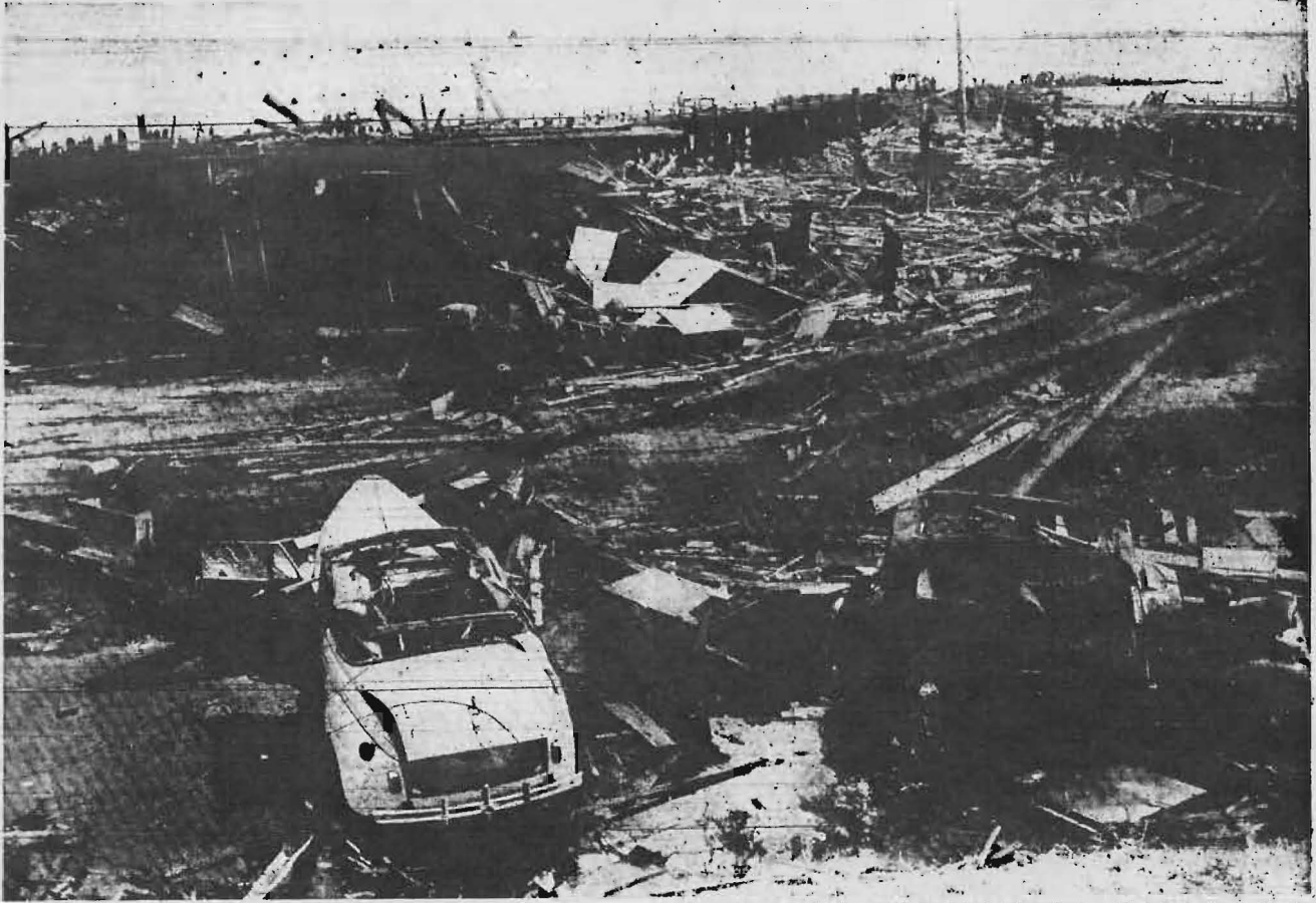
WRECKAGE —This is a general view of the enormous damage done to the dock area at Port Chicago by the explosion of the two ammunition ships. Literally blown to matchwood, the debris in the background is what was left of railroad equipment and installations. Concussion reduced the two automobiles in the foreground to little more than candidates for the junk yard.
