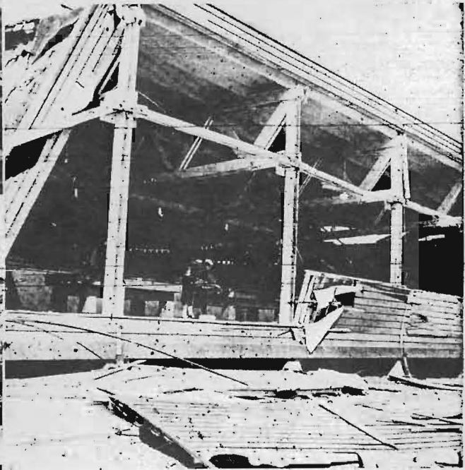
GAME GOES ON —The Navy adjusted men's recreation hall was more than a mile away from the actual explosion, yet one wall was blown completely out and another part of the building collapsed. In the above scene showing the blown-out wall, a shore policeman has nonchalantly picked up a cue and is pictured making a few practice shots on one of the pool tables.
