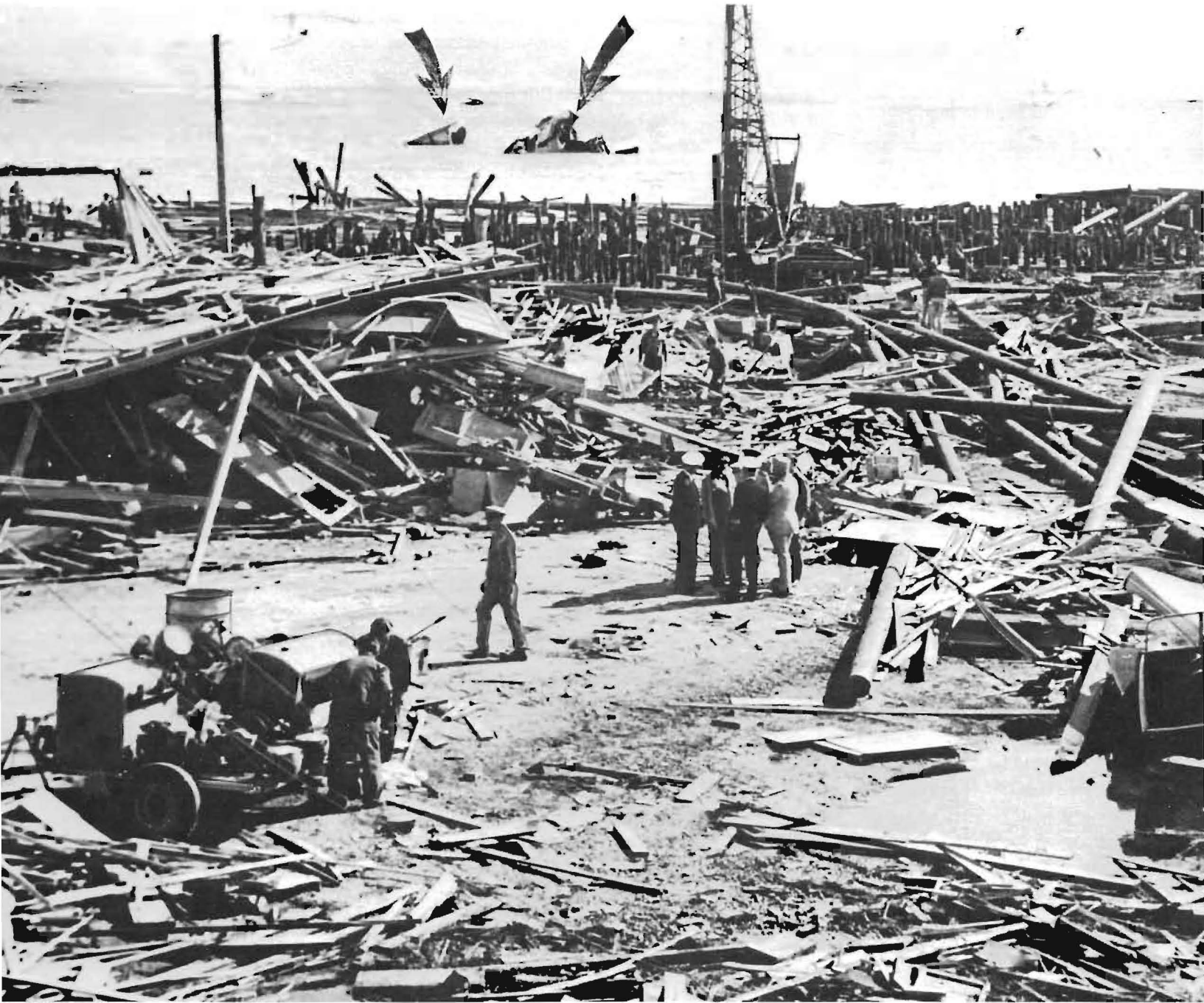
Bits of wreckage (marked by arrows) protrude from the water at Port Chicago, all that remained of the two ammunition ships which exploded. In the foreground are the shattered remnants of the dock with its railroad equipment and installations.
