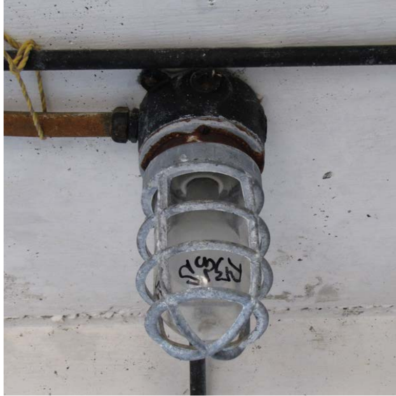
15. Sole intact light bulb housing on the ceiling of the repeater room inside B 5 S 5 Battery Townsley.
