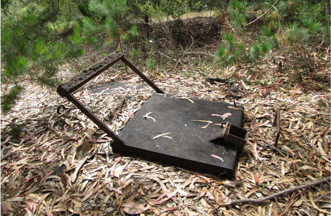
8. Sealed manhole hatch to B 8 S 8 Battery Davis. Author, July 8, 2015.
