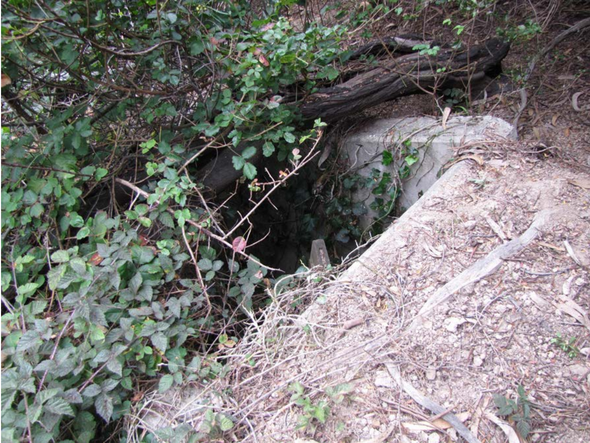
19. Dug-in entrance to power house. Author, July 8, 2015.
