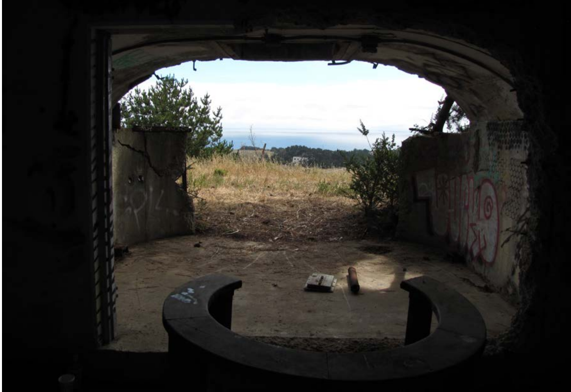
11. View from the rear repeater room with demolished interior wall inside B 5 S 5 Battery Townsley. Author, July 8, 2015.
