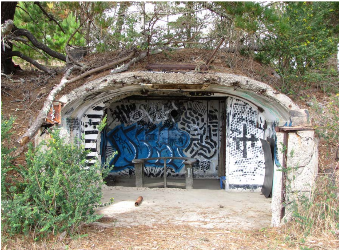
9. B 3 S 5 Battery Townsley, missing its steel dome and the front portion of the station. Author, July 8, 2015.
