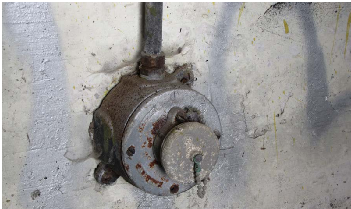
14. Pin-type electrical outlet and screw-on cover plate, on the lower right-hand portion of the rear wall to the repeater room inside B 5 S 5 Battery Townsley. Author, July 8, 2015.
