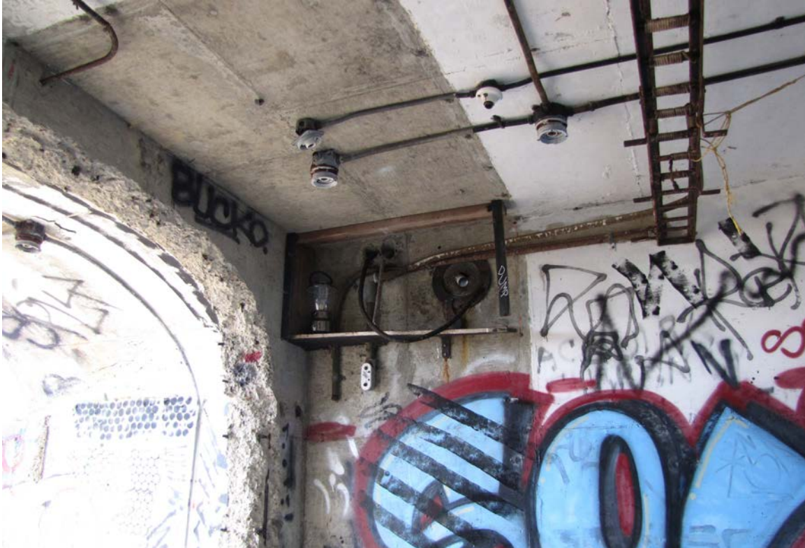
16. Light fixtures and electrical conduit on the ceiling of the rear repeater room of B 5 S 5 Battery Townsley.
