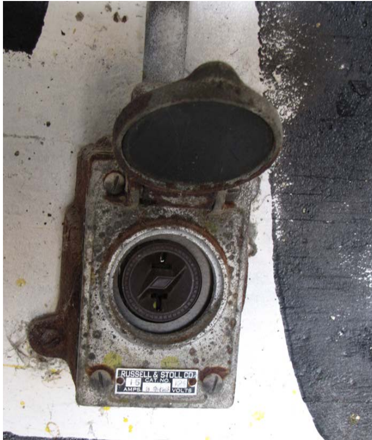
13. Standard electrical outlet plug with cover, on the rear wall of the repeater room inside B 5 S 5 Battery Townsley. Author, July 8, 2015.
