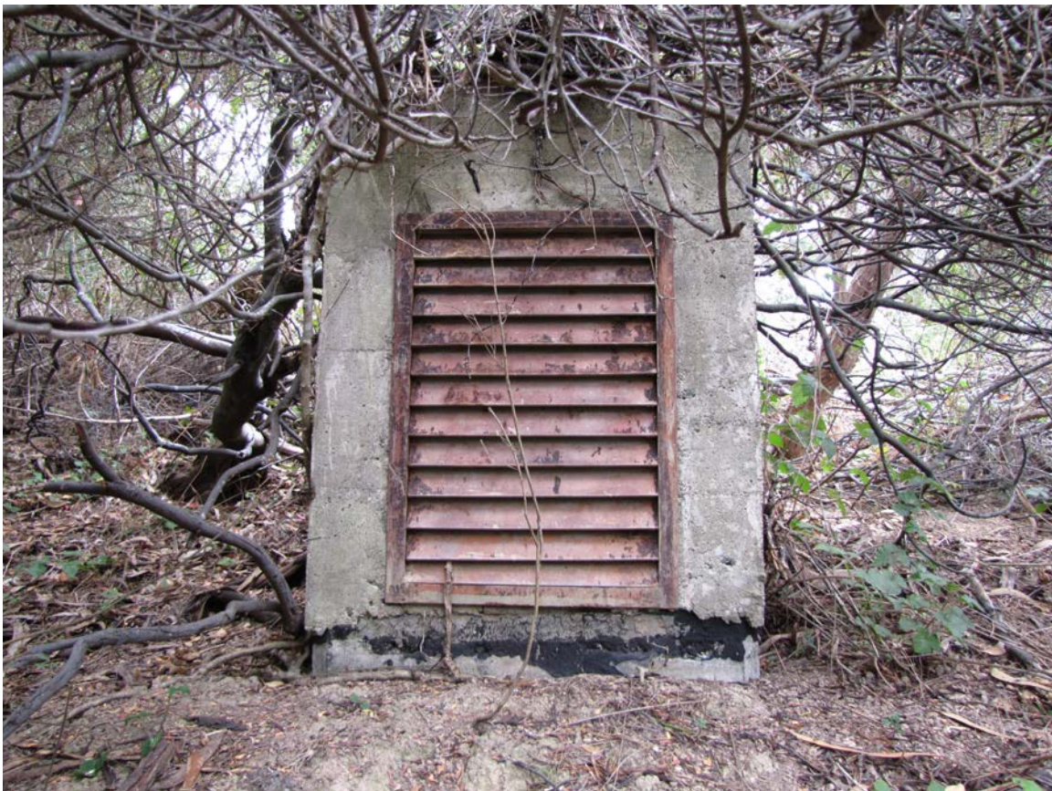
18. Vent to dug-in power house. Author, July 8, 2015
