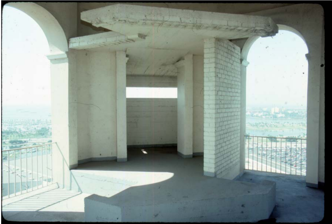
Inside the cupola fire control station 1992. Bolling Smith
