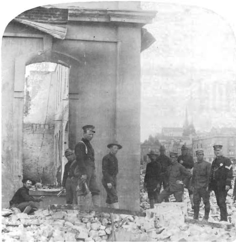
Guardsmen set sticks of dynamite to bring down dangerously tottering walls. Their seemingly random blastings during the fire did little to control the blaze and brought forth public criticism.
