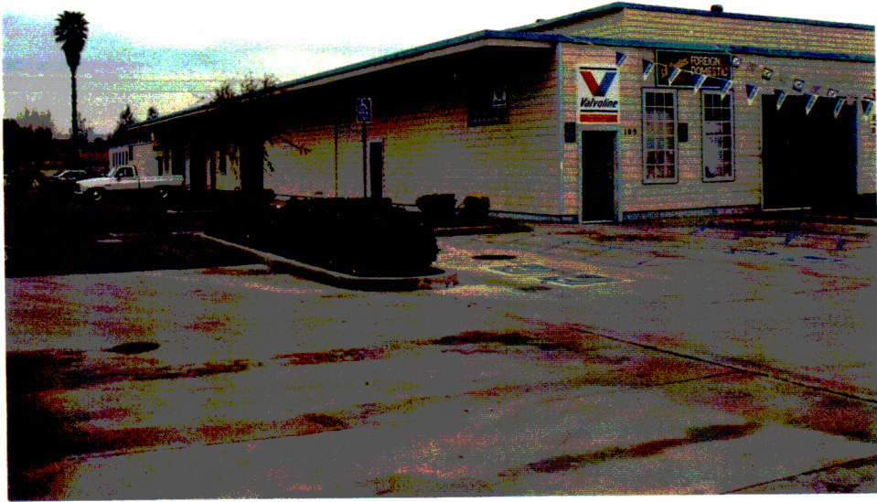
PHOTO #11 ORIGINAL BUILDING (Corner of Arlington Avenue and Rutland Avenue, Facing Northeast)
