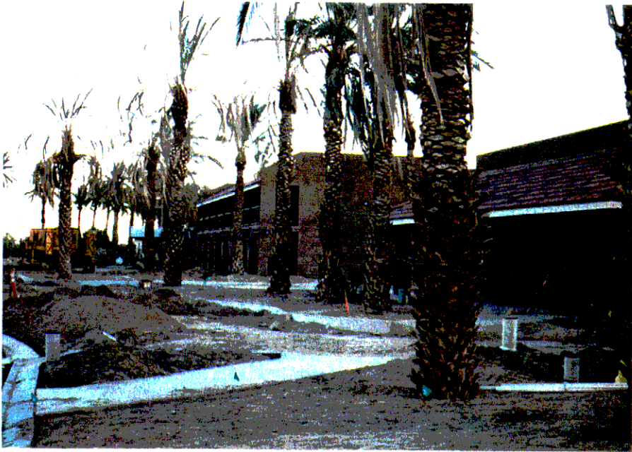
J-7 Some of the new construction that has taken place on the former Camp/Ranch Ensign.
