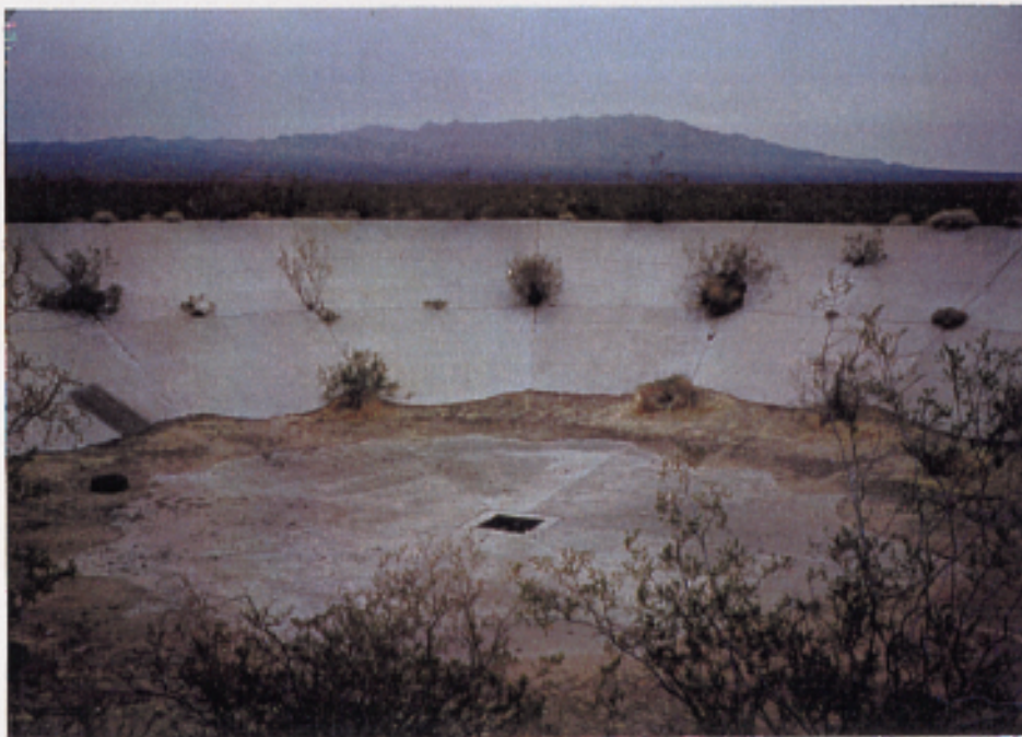
J-15 500,000 Gallon Concrete Reservoir
