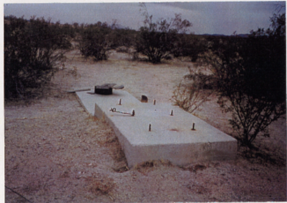
J-16 Abandoned Well Located Near Reservoir
