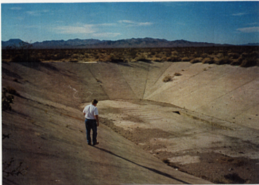
J-3 Looking S, 50,000 gal. water reservoir.
