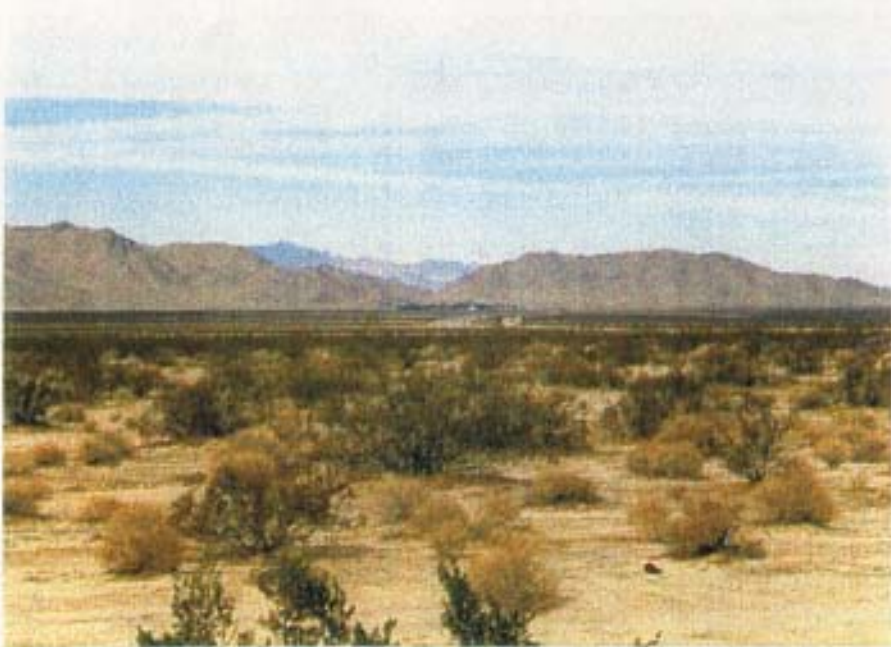
J-11. View north towards the water pumping station.
