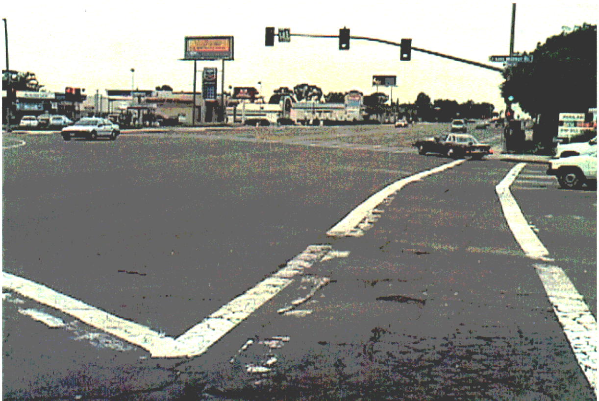
J-10. Area C: Intersection of Navajo Road and Murray Blvd.
