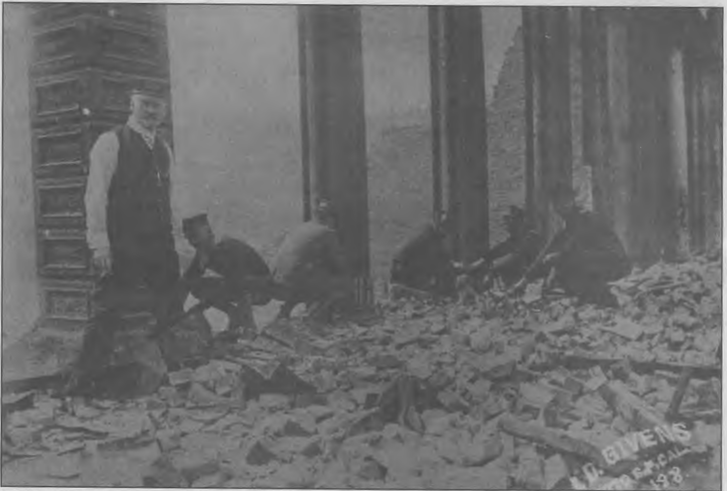
Figure 11: A six-man dynamite squad at work in the post-earthquake rubble of San Francisco during the great fires of April 18-21, 1906. This squad consists of a San Francisco City Police officer (left), possibly Sergeant J.H. Morrissey, four U.S. Army Regulars, and a single civilian (right). Note the dynamite sticks being secured to columns at center. Photo (#188) by James D. Givens, originally published on page 48 of his 1906 "San Francisco In Ruins" Photo-Essay, with the caption: "Dynamiting Crew of Regulars Destroying Buildings to Retard the Progress of the Flames." California Historical Society/University of California, Berkeley, Bancroft Library.
