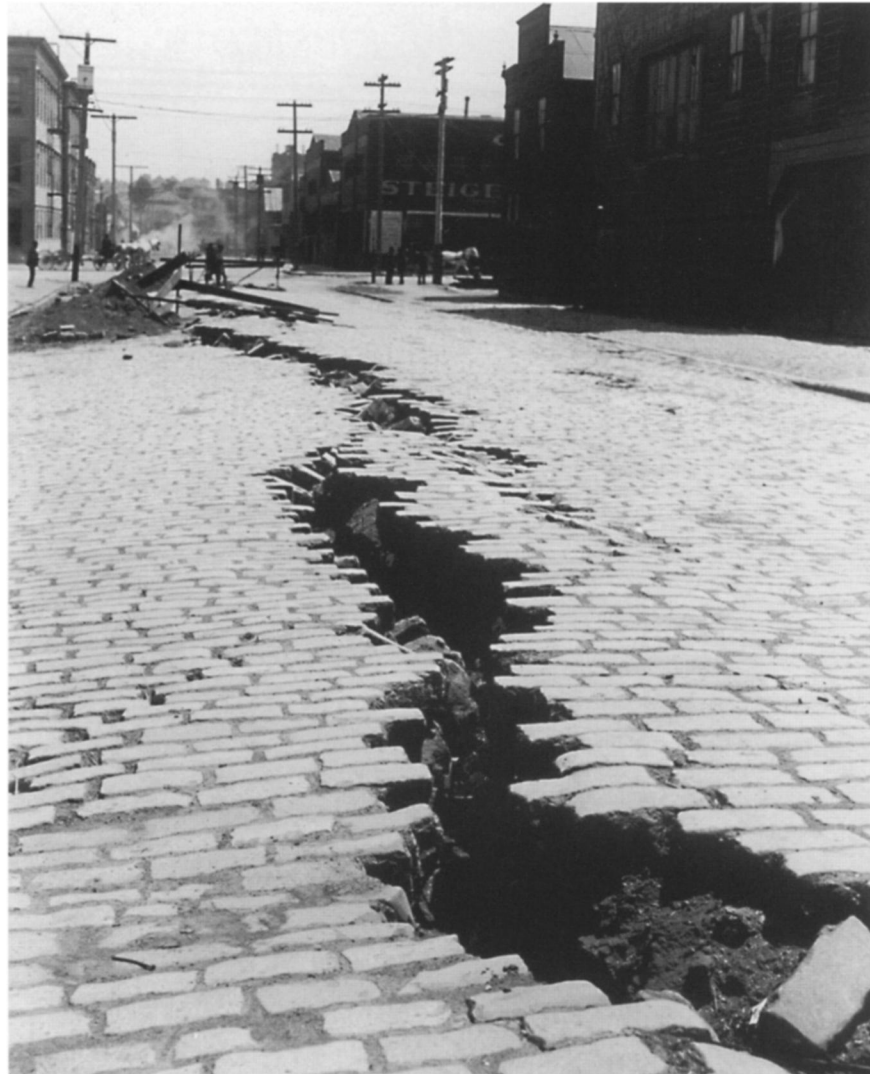
Crack in the Street Folsom Street, San Francisco CALIFORNIA HISTORICAL SOCIETY, FN 26472
