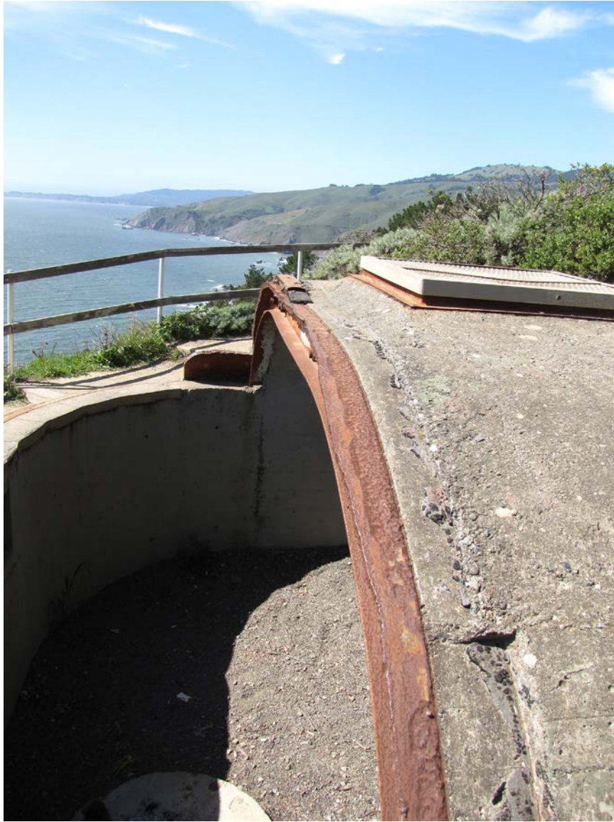
8. Evidence of cutting torch use. B 2 S 2 Battery Smith/Gutherie with remaining portion of steel dome attached to the roof of the station. All photos are by author, April 4, 2016.
