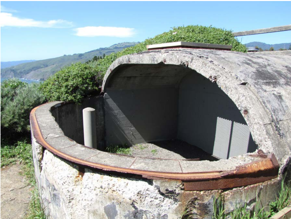
11. B 4 S 4 Battery Wallace with pipe pedestal mount.
