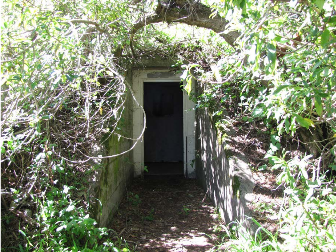
14. Entrance to the dug-in power house.
