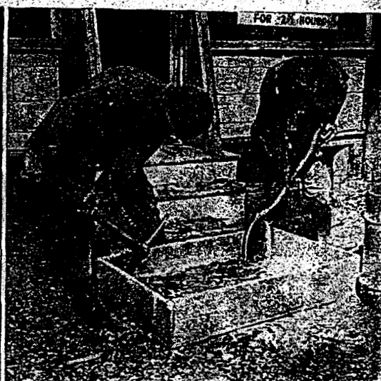
Figure 23. Dry mix of earth and bleach is prepared in shuffle box.
