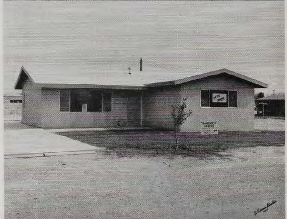
INDIO Progress—one hundred and twenty-nine homes were built in the Coachella Valley by Thunderbird Homes in 1957. Top photo shows typical three bedroom, two-bath home. Bottom photo is typical three-bedroom, one-bath structure. The popularity of these homes is such that Thunderbird Homes has established branches in Riverside and an Bernardino.
