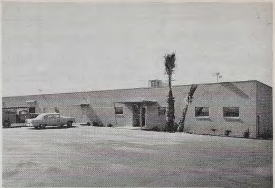
RECENTLY completed Service Center of California Electric Power Co at Apple Valley. Center houses warehouse, construction and operating personnel and facilities.
