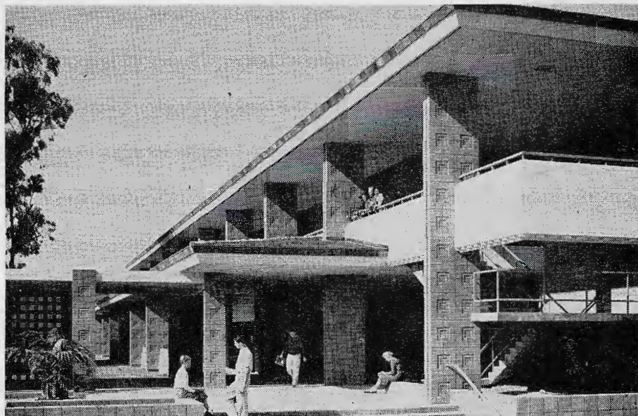
—Photo Courtesy H & H Roofing Co NEW Music Building at University of California, Santa Barbara College, showing predominant architectural style on this 408-acre ocean front campus.
