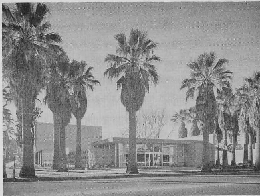
ATTRACTIVE new Security First National Bank building in Hemet gives an indication of the vast banking house's faith in the lovely Hemet-San Jacinto Valley.
