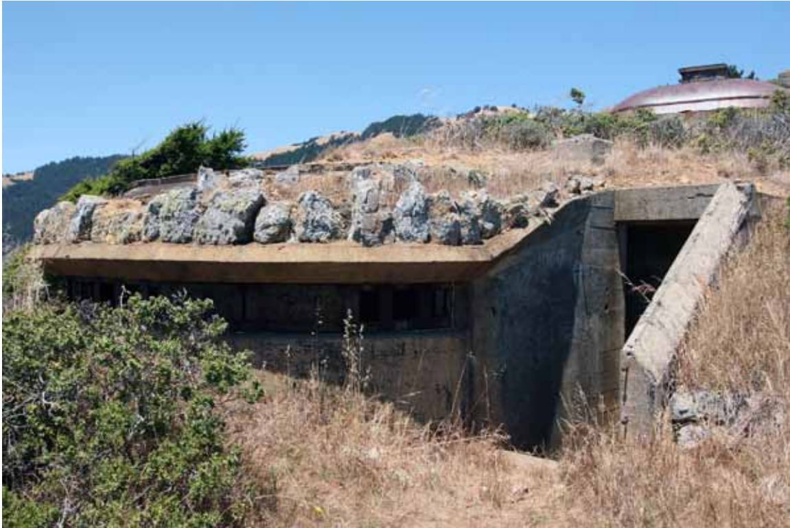
B 6 S 6 129, Hill 640; current condition illustrates side entrance. B 3 S 3 129 is visible above the lower station.
