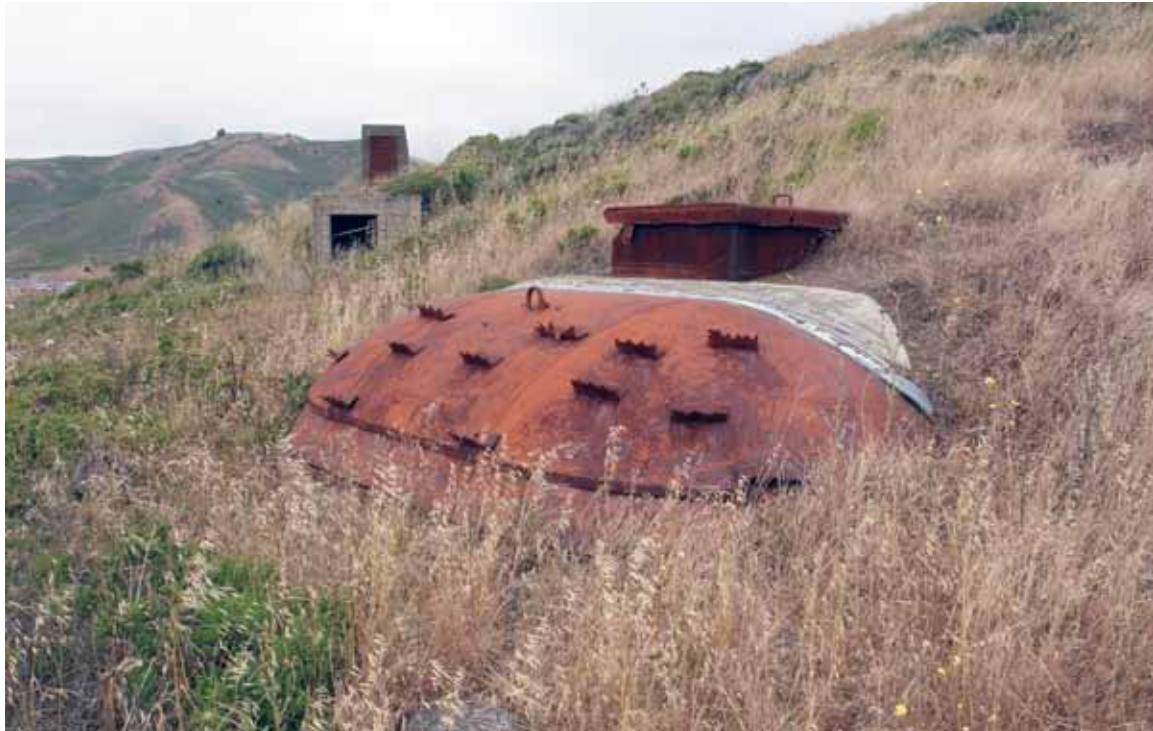
BC Wallace, showing bracket for attaching rocks for camouflage. John Martini
