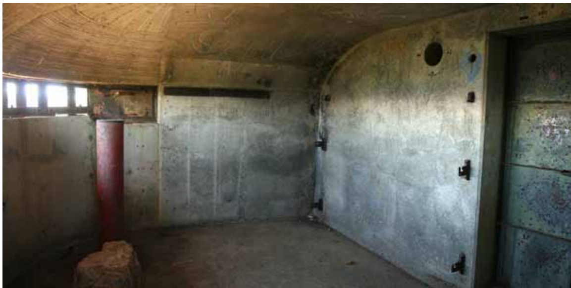
B 6 S 6 129; current condition of interior. John Martini
