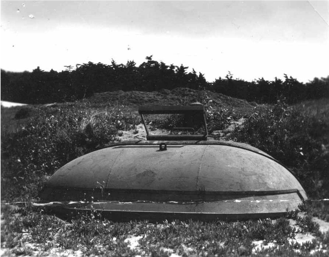
Wartime photograph of unidentified domed fire control station, showing exterior counterbalance that was the subject of complaint. NARA .
