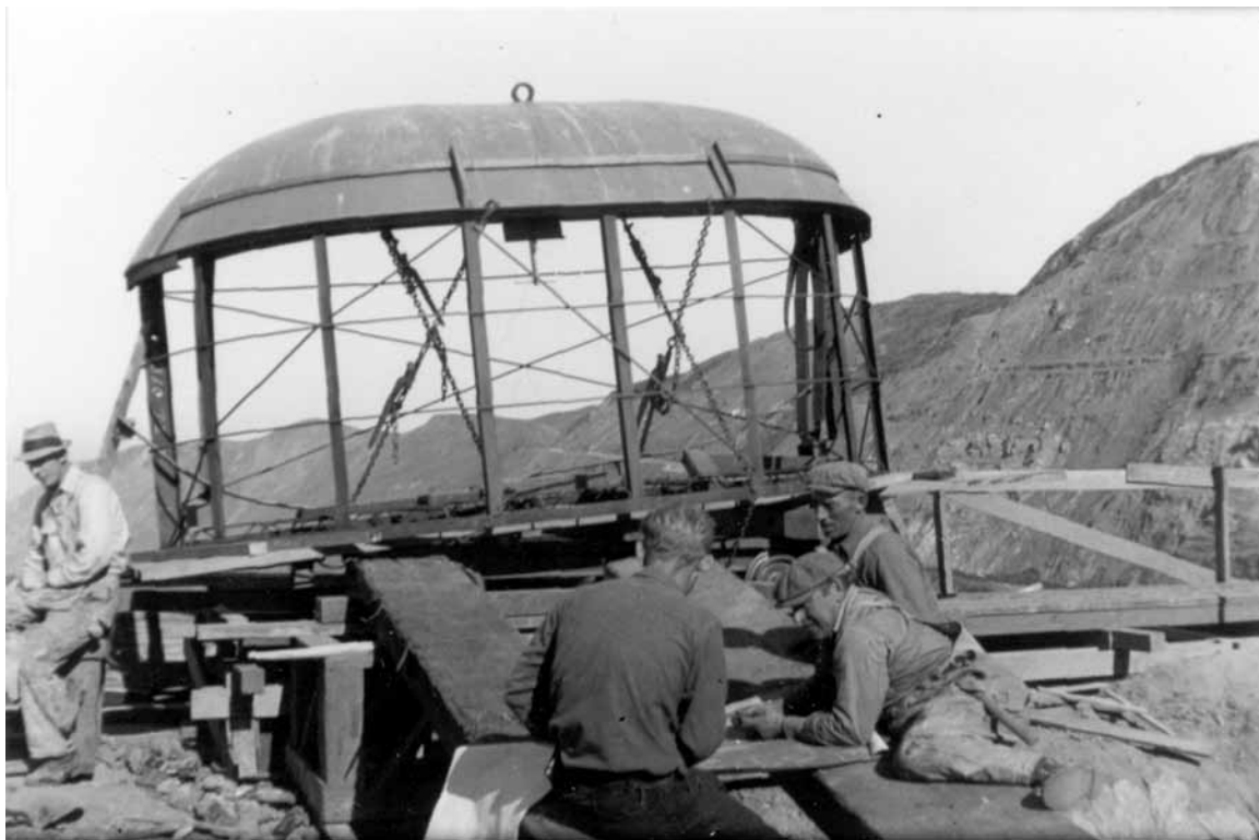
Construction of Devil's Slide domed station. E.R. Lewis Collection
