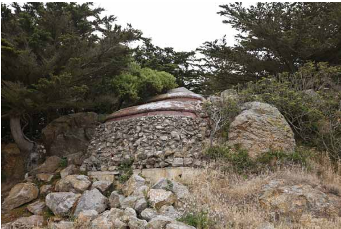
Sutro Heights FC stations. Rocks remain attached to the lower part of the steel, while those once attached to the actual steel-dome roof have been removed. John Martini
