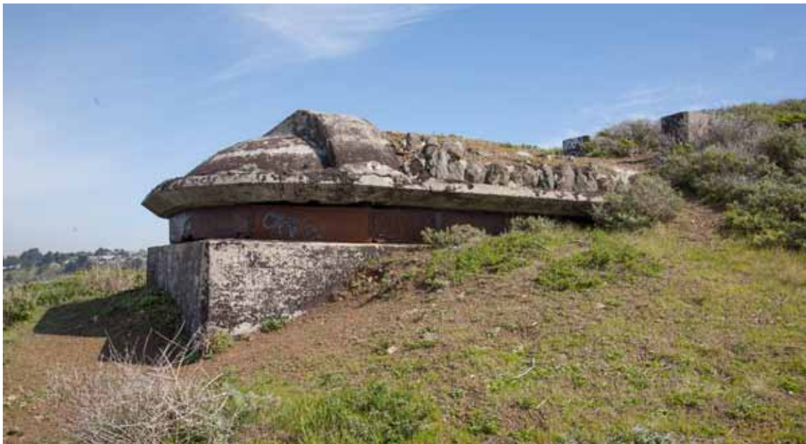
BC Battery 244, showing rocks still attached to rear roof and the lip where rocks were once attached to front of domed roof. John Martini
