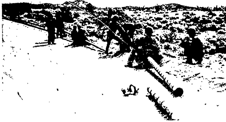
Four-man coupling crews at work putting in a portable pipe line. This pipe line went over a rise and down to water storage tanks of the Santa Fe Railroad, a distance of seven miles. (From the files of the Engineer Board, Yuma Test Branch)
