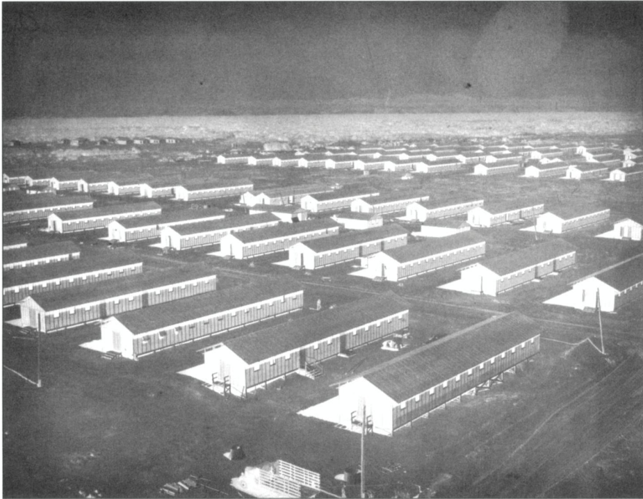
Living quarters of the Japanese American evacuees at the Colorado River (Poston) Relocation Center, Arizona. Fred Clark, photographer. National Archives (210-g-a190).
