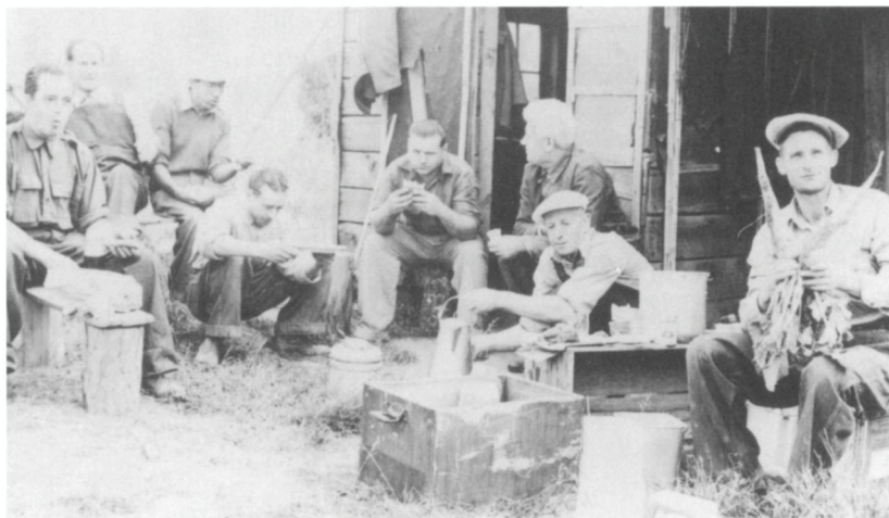
The many internees who had been granted work paroles were employed in downtown Missoula, on railroad lines, on farms, in hospitals and with forest service crews. Italian internees pictured above take a lunch break from harvesting sugar beets.
