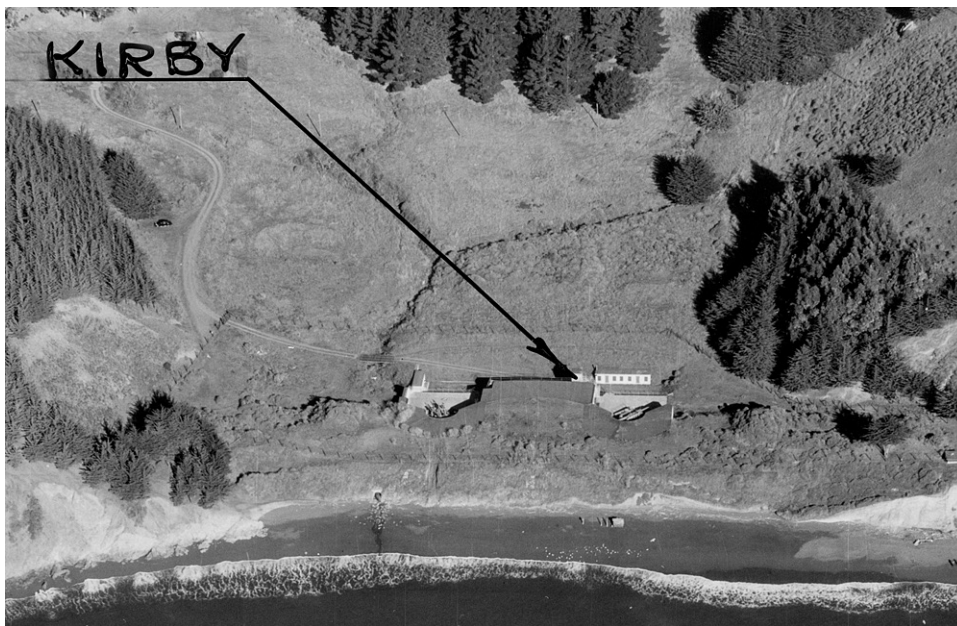
Figure 13. Oblique view of Battery Kirby, January 1938. Now-vanished features include a post-and-wire fence enclosing the battery and 1870s traverses, the road terminating in the battery parade, the latrine (left), and the guardroom/storeroom (right) behind the battery. At extreme right, a square-roofed fire control station assigned to Battery Spencer can be seen on the bluff. RG 499, E118, NARA.
