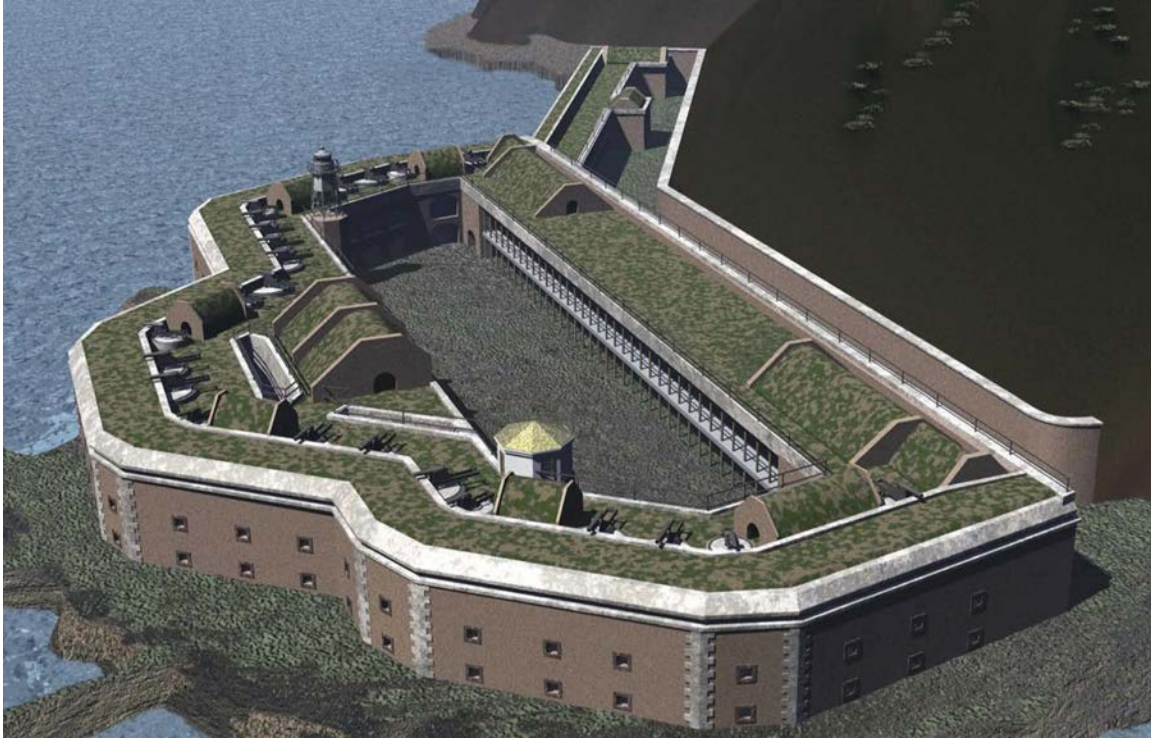
Figure 2. Had it been built, the proposed Lime Point fort would have been exactly where the north tower of the Golden Gate Bridge now rises. This artist's recreation is based on engineer plans approved in 1867. Courtesy Larry Ormsby, from Fort Baker through the Years.
