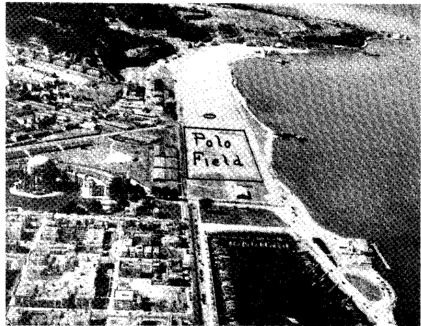
Even after the airbase was expanded to its full extent in 1926, the area east of the circle was only used by aircraft in emergencies. The area west of the circle was approximately 3,500 feet in length. (National Archives)
