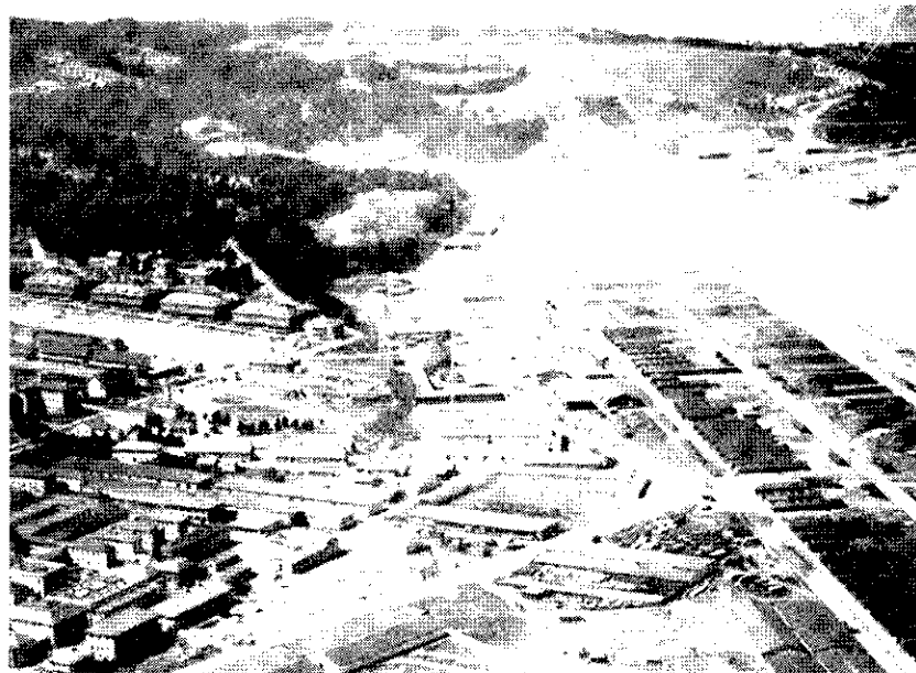
Crissy Field looking west. This photograph shows the ruts by the airmail and reserve hangars and the damage to the western portion of the field caused by taxiing aircraft. April 20, 1923. Compare this photograph to the one on page 21. (National Archives)
