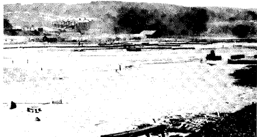
The original sand dunes and main estuarine channel through the lower Presidio wetlands just prior to their being filled. Note the Montgomery Street barracks in the background and the sections of pipe laid out prior to their being connected to the dredge. Ca. 1912. (San Francisco Public Library)
