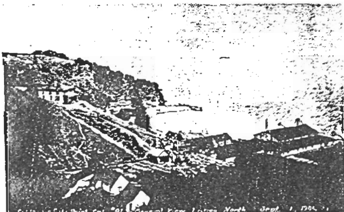
General view of the cove (looking north) during early construction of the Navy Coaling Station, Sept. 1, 1906 (courtesy Navy Dept., National Archives).
