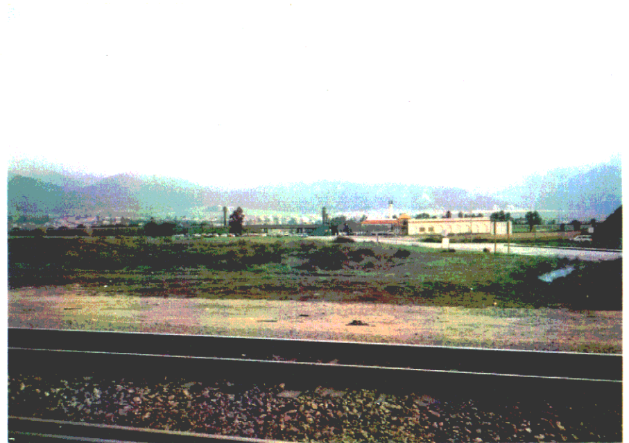
J-4 View of Area C from northeast to southwest.
