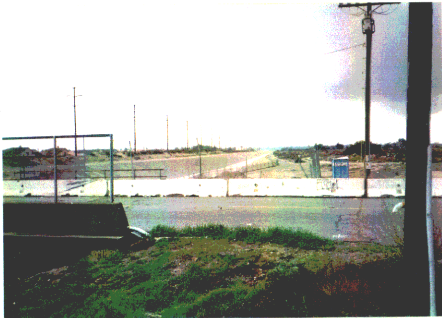
J-11 Drainage Ditch, view south.
