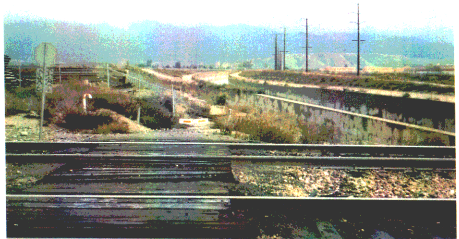
J-12 Drainage Ditch, view north.
