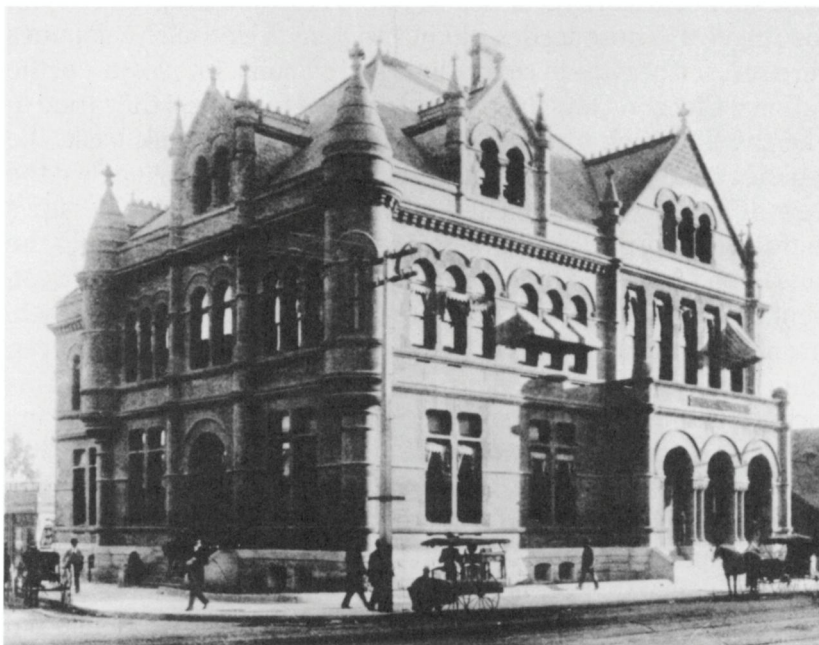
The Los Angeles Federal Building at the corner of Main and Winston. It housed the Federal District Court where the Grand Jury prepared indictments against the local ARU leadership. Courtesy Security Pacific Collection/ Los Angeles Public Library.
