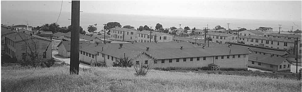
WW I Barracks area, Angels Gate Park 1991 (photo by Mark Berhow)
