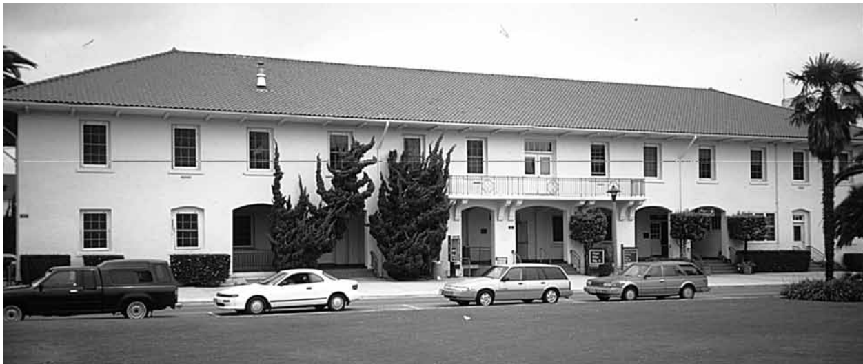
Barracks, Middle Reservation, Fort MacArthur 1996 (photo by Mark Berhow)
