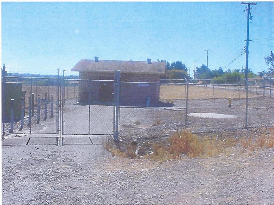
K-15 Pumping Station on 8.68-acre parcel.
