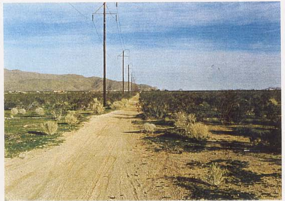
J-2 (Area A) Looking east from the center of the target area.
