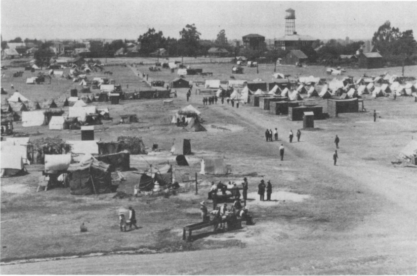
Looking west from a barn roof toward the town of Wheatland, this photograph captures mid-day activities at the Durst hop pickers camp. Wheatland Historical Society. C. C. Green photograph?
