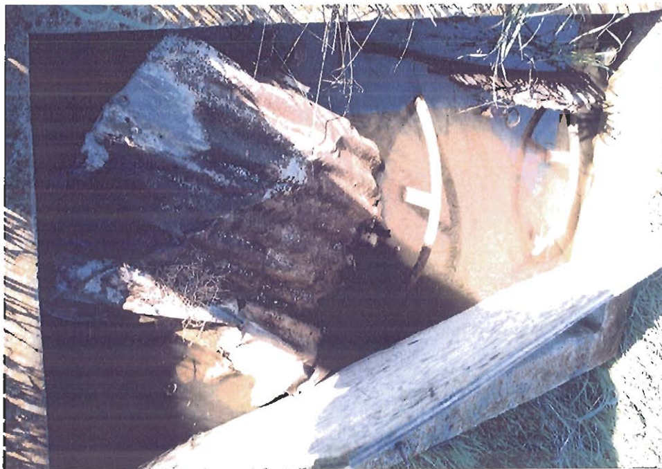
Photo #4 Former FUDS fire water supply concrete pit
