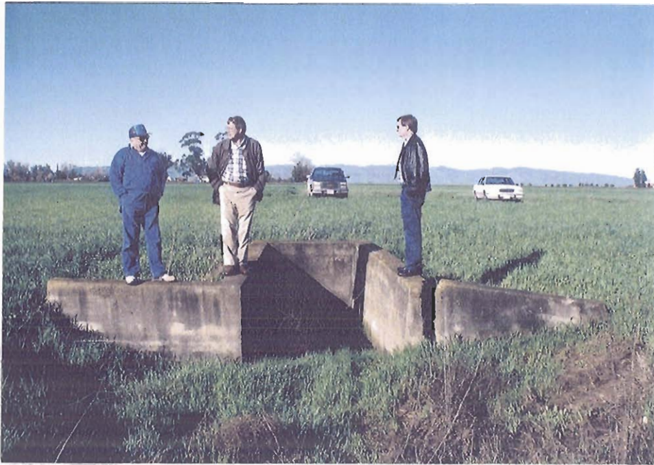
Photo #5 Tunnels under runways/taxiways turned out to be drainage structures with wing walls
