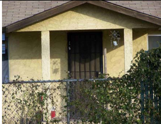
Figure 33: View looking southeast at the newer exterior surface of 8650 Cypress Avenue
