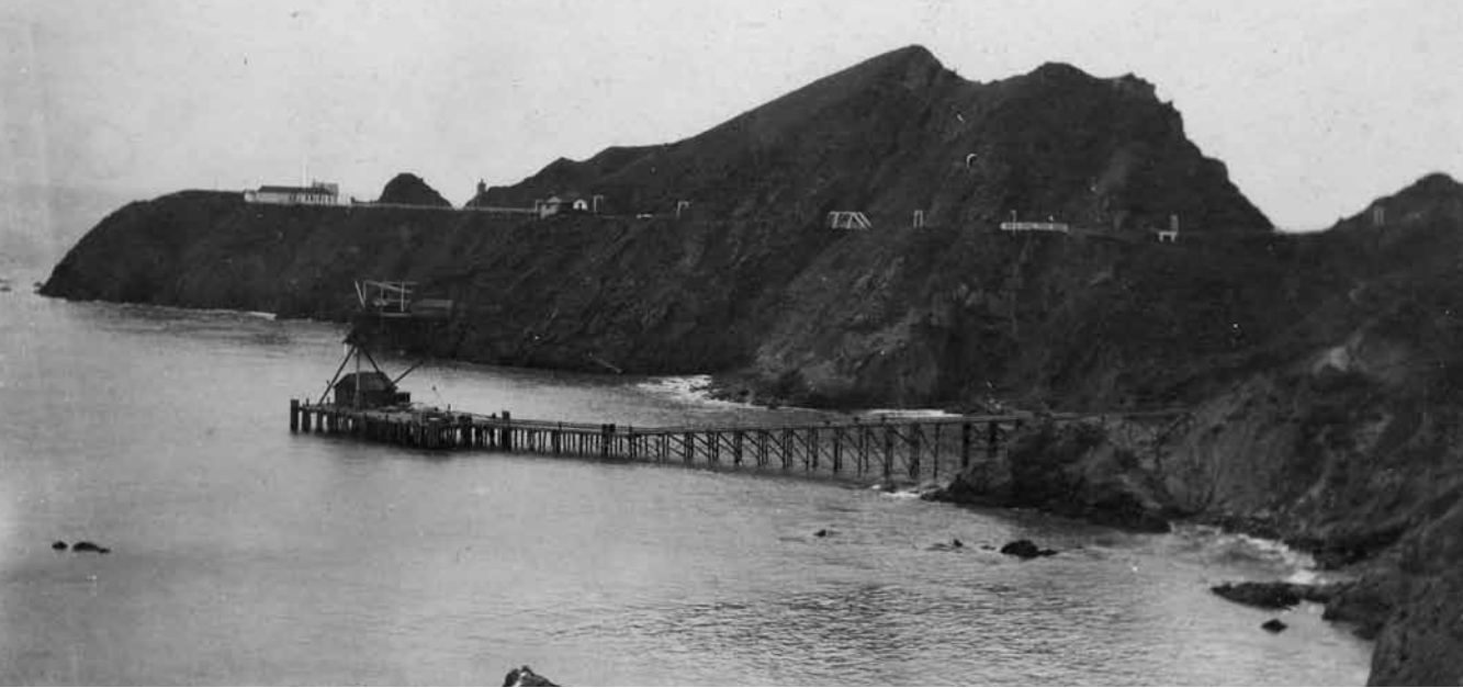
Above: A view of the engineers' wharf and trestle down at Bonita Cove, as well as the tunnels and walkways leading to the Point Bonita Lighthouse in the background. (Photo circa 1915)
