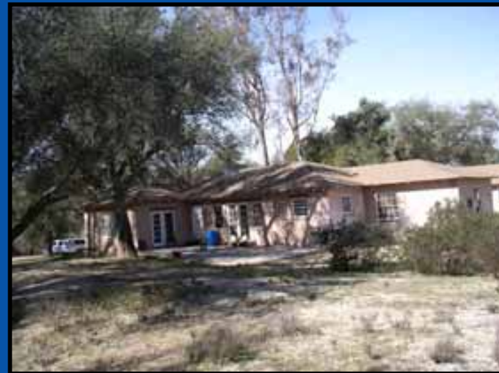
Ferguson Ranch House used for tactical Headquarters
