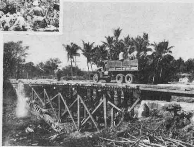
RIGHT: BRIDGE BUILT ON FOUND- ATION OF FORMER BRIDGE
