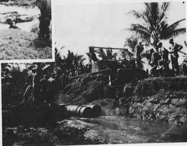
RIGHT: 55 GAL DRUMS USED AS CULVERTS
