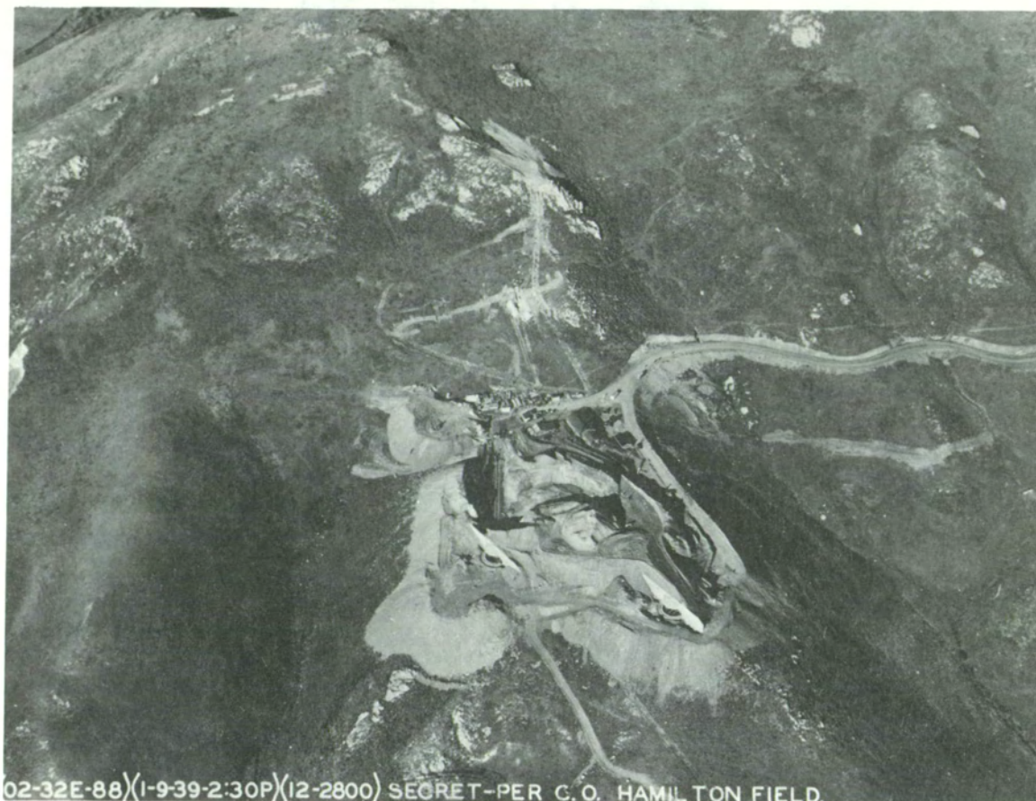
17. Battery Townsley nearing completion, Fort Cronkhite, 1939.
