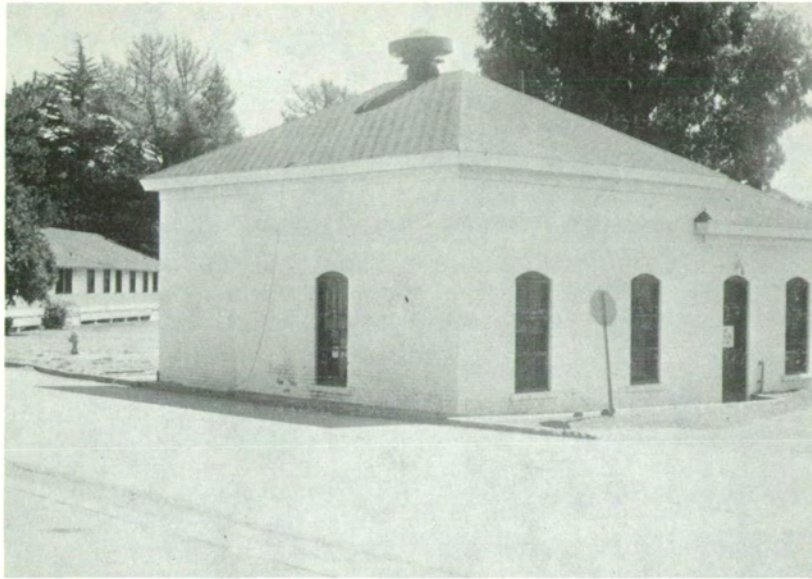
7. Pumphouse, Fort Baker, 1977.
