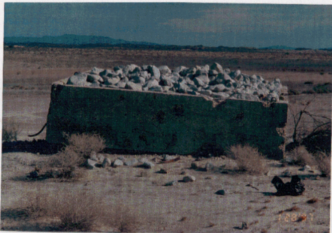
J-7. Area E-1 (Borrego Wash): One of Two Collapsed Rake Stations.
