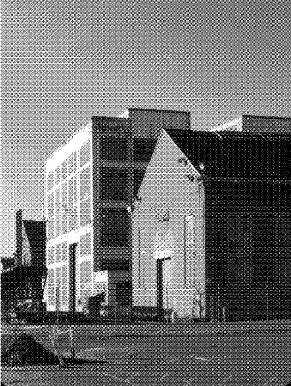
Figure 17. Building 271 at Mare Island, 1918. The glass-enclosed curtain wall building is at the center. Although it was a thoroughly modern industrial building for its time, it was integrated structurally with 19th century brick buildings. (Source: Historic American Buildings Survey, photographer William Dewey.)
