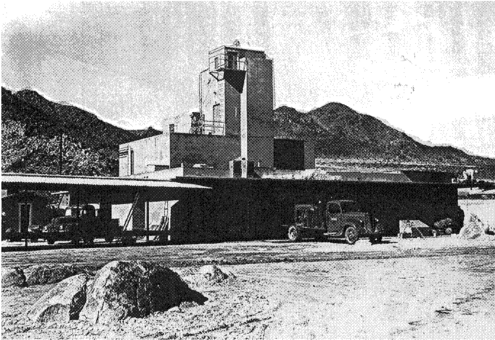
Figure 29. Press Building at NOTS Inyokern (now NAWS China Lake), November 1944. This building epitomizes the dictum "form follows function"; its sculptural form is simply the shape of the reinforced concrete needed to encase machinery to press propellant grains into rocket motors. These motors were used for test purposes and in rockets used by the Navy in Europe and the Pacific. (Source: The National Archives.)
