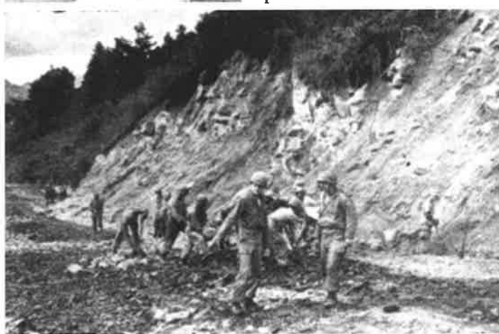
GOODBYE MUD-Members of the 578th Engineer Battalion work on one of the mountain roads, filling it with rocks in their fight against mud. They were responsible for building countless miles of road to keep the division moving as easily as possible.
