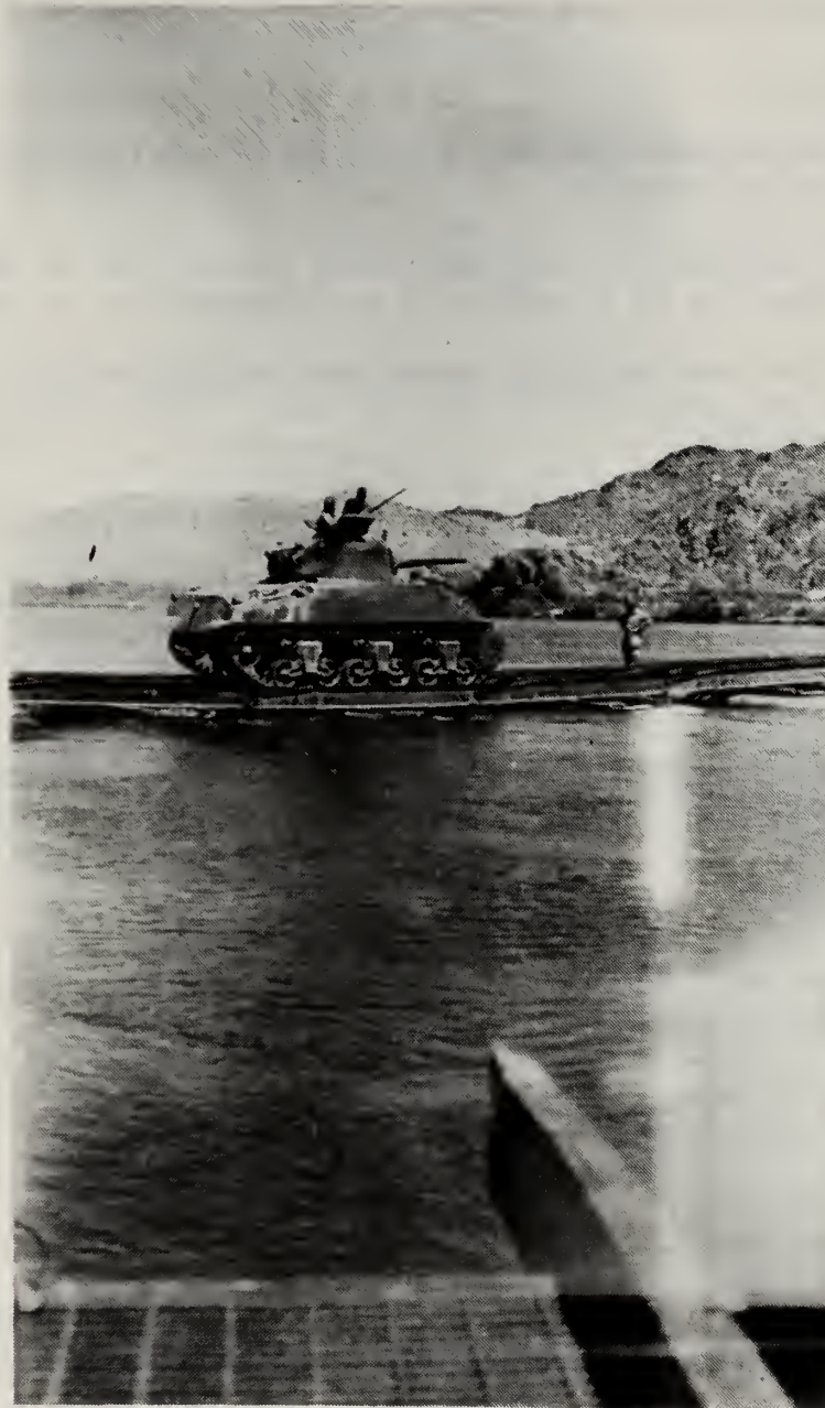
Here, a tank crosses the Colorado River on pontoon bridges (also seen in foreground)
