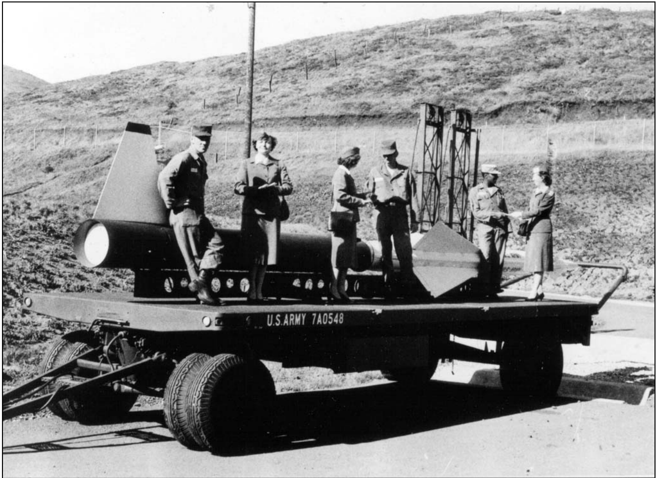
The same group of soldiers and Red Cross workers atop a Nike-Ajax transport trailer, parked at the fueling area. In the background are the two fueling towers for hoisting barrels of red-fuming nitric acid and oxidizer. (Golden Gate National Recreation Area, Henry E. Paine Collection)
