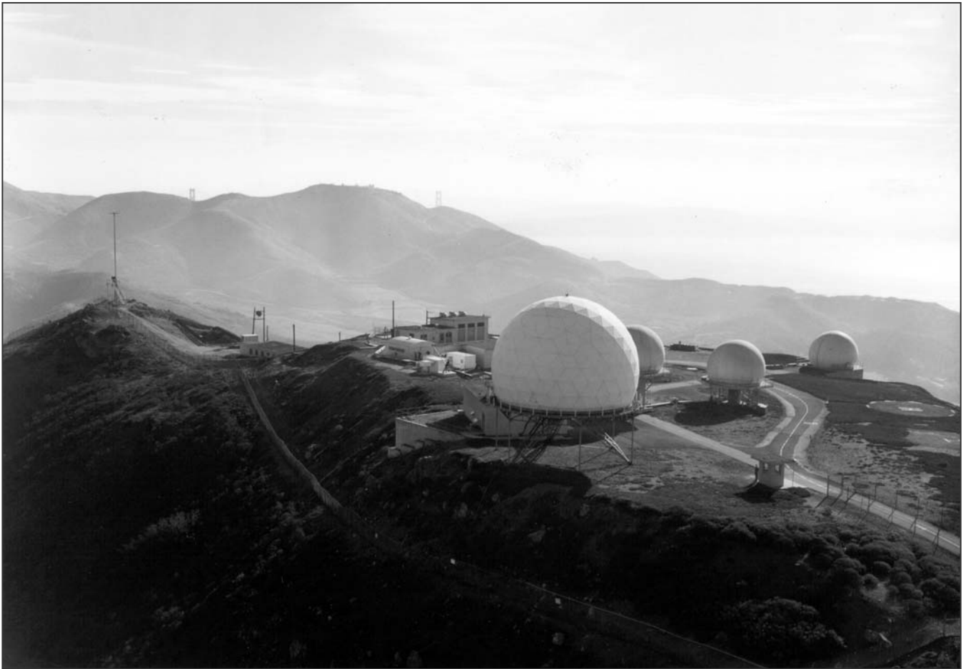
Integrated Fire Control (IFC) site SF-88C about 1970. The large dome at center shelters the HIPAR (High Power Acquisition Radar), while the smaller domes cover, from left to right, the TTR (Target Tracking Radar), TRR (Target Ranging Radar) and MTR (Missile Tracking Radar). On the knob at the far left is the bore-sighting mast. Following the Army's departure, this location came to be known unofficially as "Hill 88." (Golden Gate National Recreation Area, TASC Collection)
