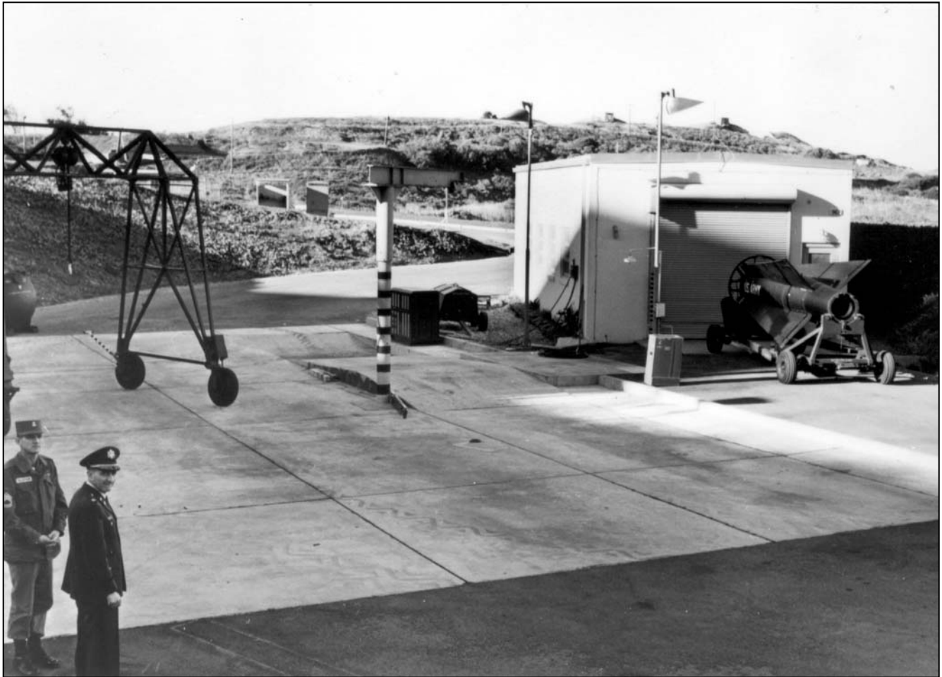
Fueling station in 1961, with “A-frame” portable hoisting unit at left and a Nike Hercules forward body section next to the Warheading Building at the right. In the background are the former Acid Storage Shed, now converted to a flammable materials storage building, and a portable latrine. U.S. Army photograph.
