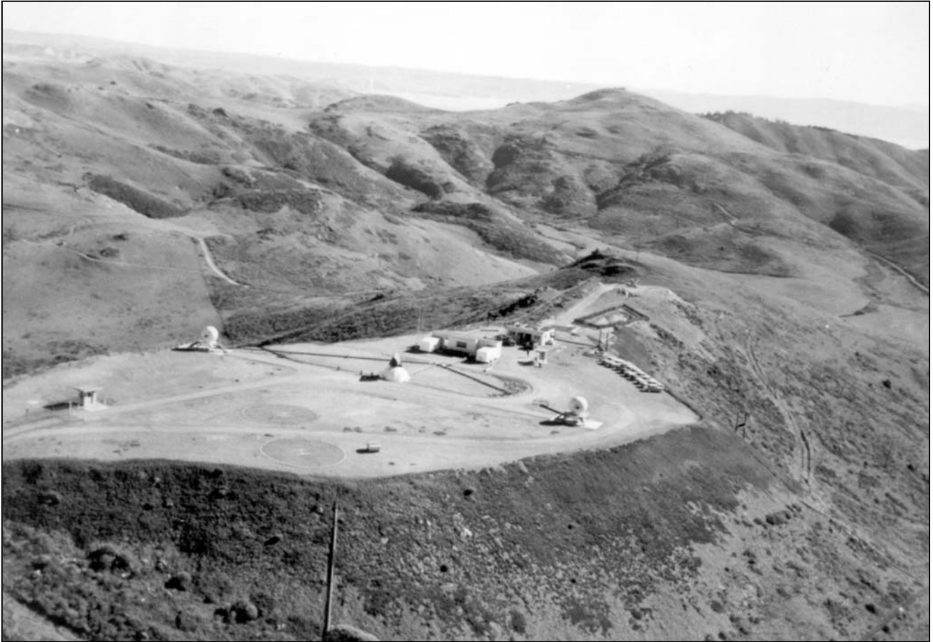
SF-88C in its original configuration, October 2, 1959, before the large HIPAR dome was installed. From left to right are the TTR, the low power acquisition radar (LOPAR), and the MTR Behind the acquisition radar are the battery control and radar control vans, joined by a concrete connecting corridor building, and the generator building. (Golden Gate National Recreation Area, DOD Still Media Records Center Collection)
