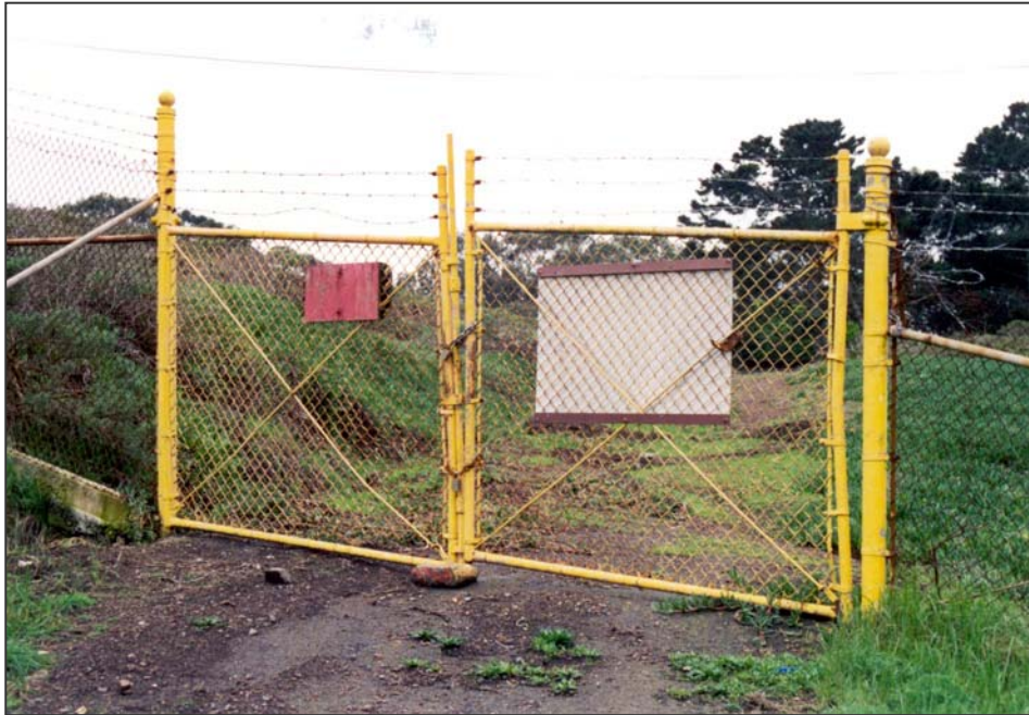
Gate in “Limited Area” fence leading to Battery Alexander
